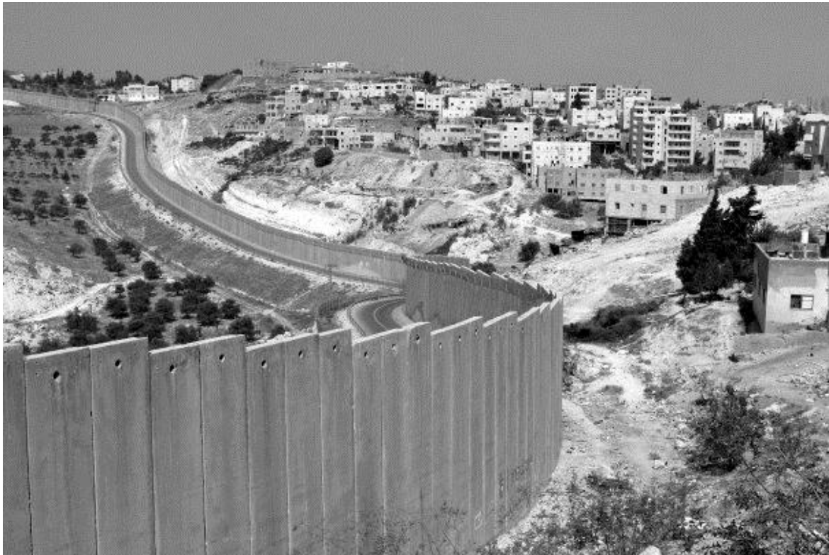
The Israeli wall is to 85% built illegally inside the occupied Palestinian territory, dividing Palestinians from Palestinians. Photo: Aida-Burnett Cargill
